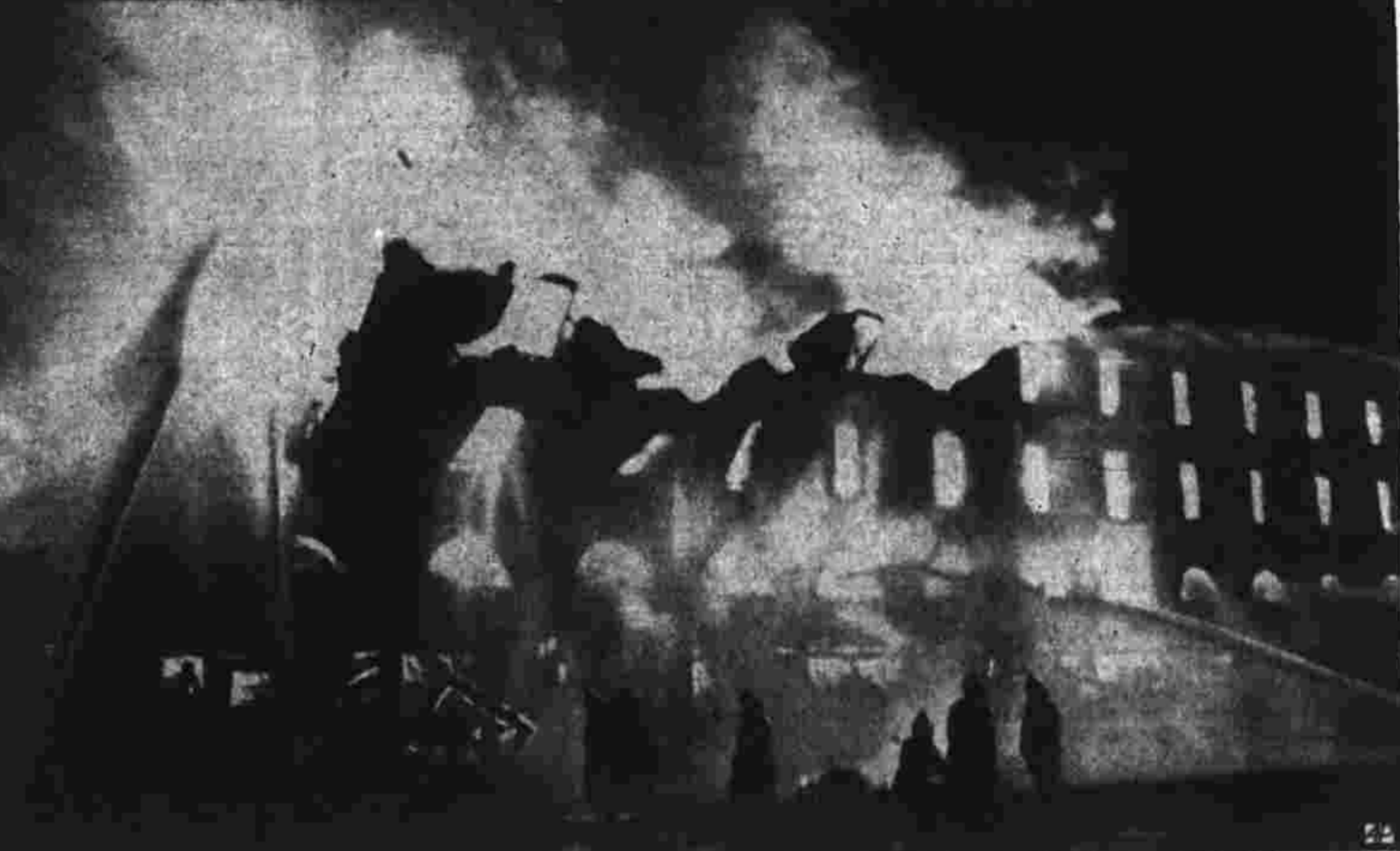
One of the walls of Bienville Warehouse Corporation in New Orleans, La., is shown collapsing during the fire which ravaged the block-square building and caused an estimated $3,000,000 property loss. Eighteen firemen were injured, some by falling walls, in what was described as the city's worst decade fire of 20 years. The warehouse was well filled with foodstuffs and cylinders of gas used in air conditioning. Bulk of the loss was in sugar, neighboring warehouse men estimating that nearly 2,000,000 sacks were stored in the structure.
